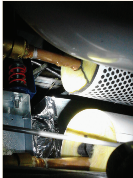
PHOTO 9 Incomplete insulation installed without enhanced quality control.
