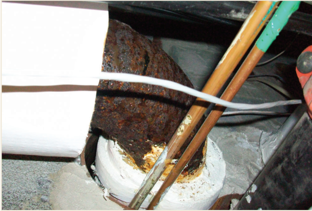
PHOTO 1 Pipe section left unsealed.
