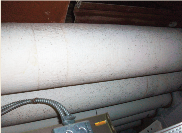
PHOTO 6 Mold spotting caused by excessive humidity.
