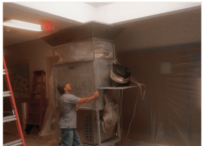
PHOTO 8 Insulation removal using portable hood.
