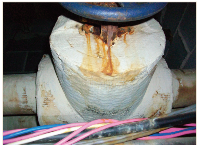
PHOTO 5 Minor water damage.
