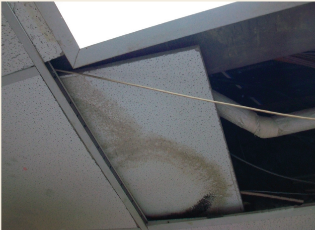
PHOTO 3 Stained ceiling tile under sweating chilled water pipe.
