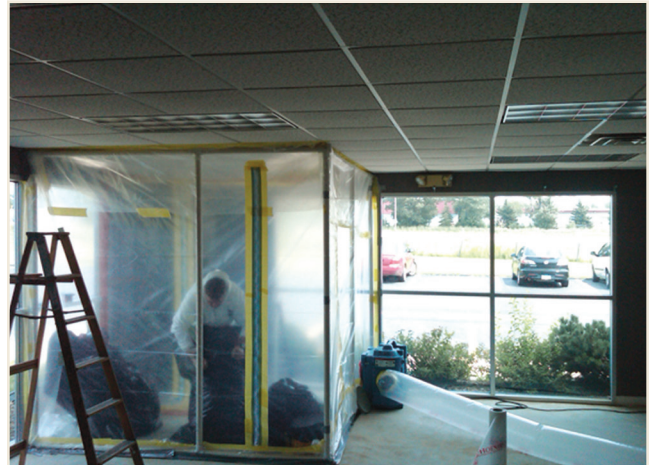
PHOTO 7 Insulation removal following hazardous material procedure.
